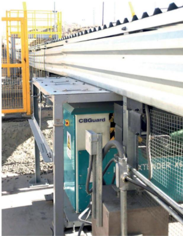
Figure 1. A CBGuard Life Extender in an overland conveyor.
